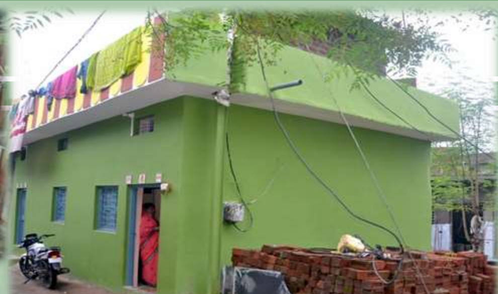
Completed BLC DUs in Hoshangabad
