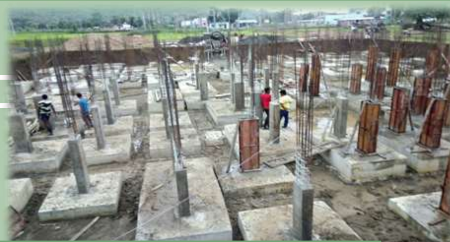
Under Construction AHP DUs in Sarni
