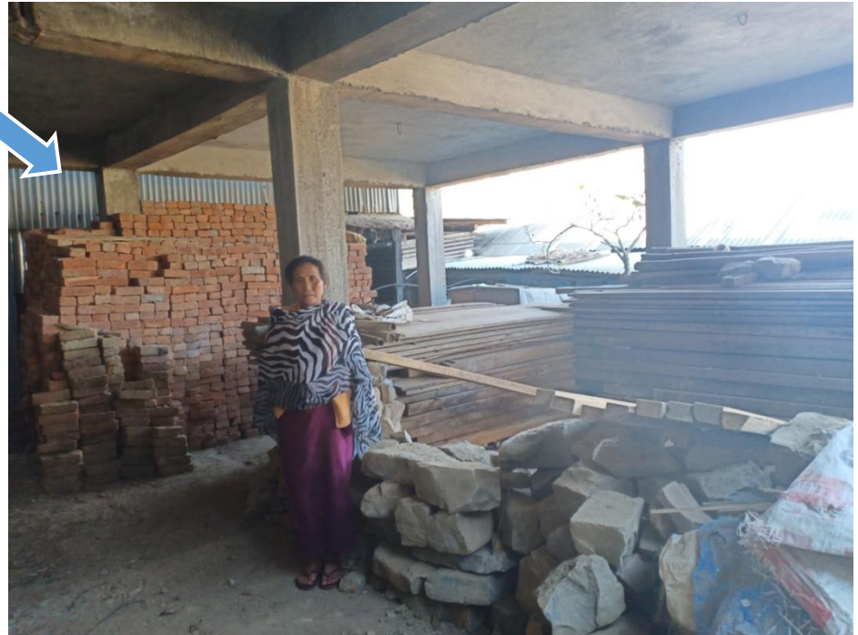
Under BLC - New House Construction in Kohima Town
