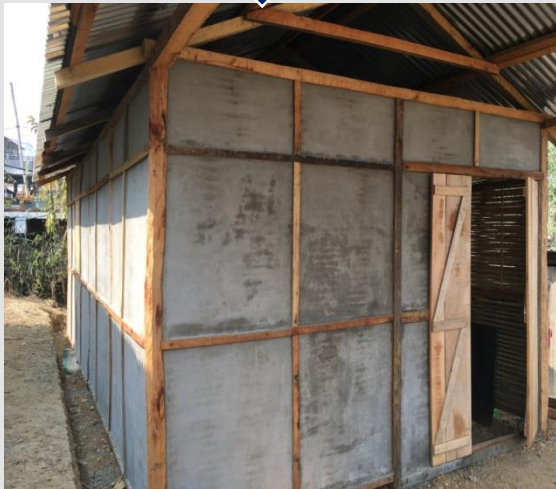
Cement Plaster on Bamboo Split
