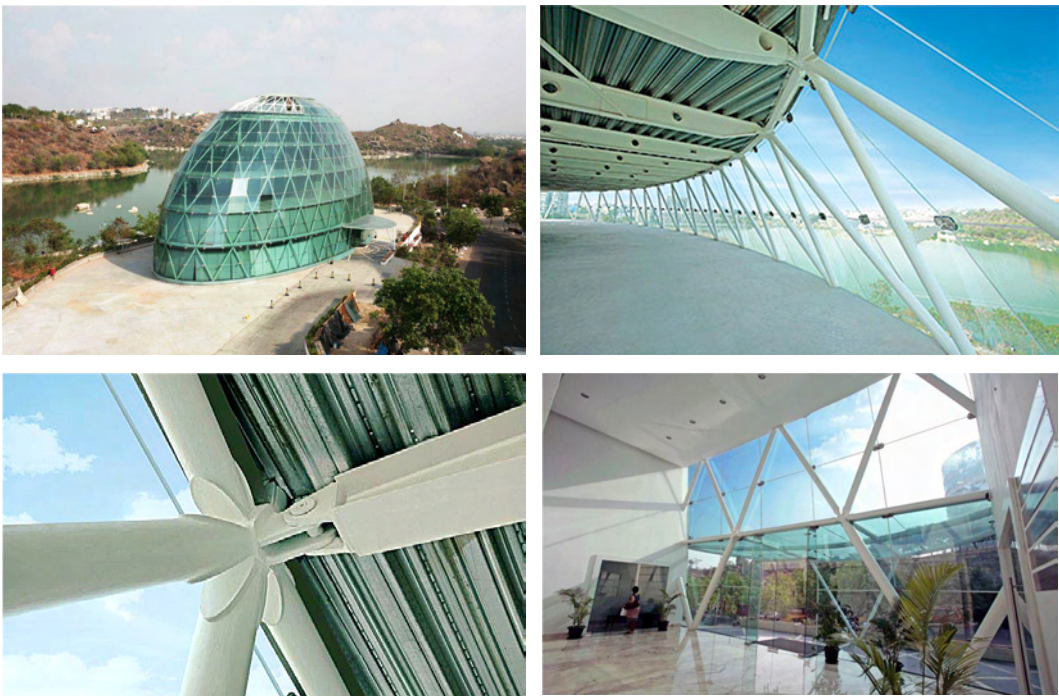
Fig. 6.15: Views of different parts of the building
