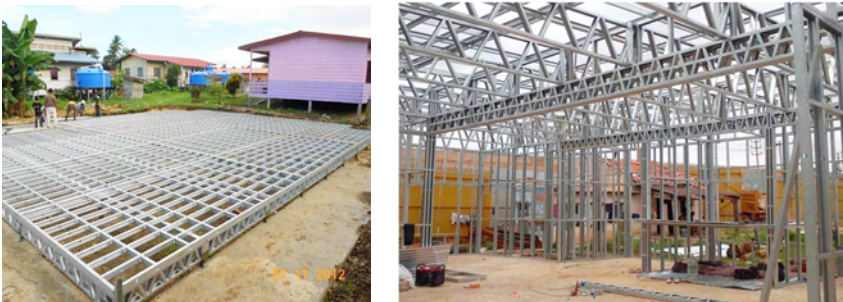
Fig. 6.4(e): Flat roof components in LGSF
