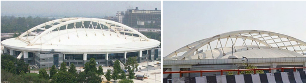
Fig. 6.13: View of the massive roof structure
