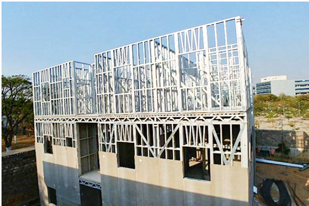
Fig. 6.13: Installation of sheathing boards (external cover) over LGSF frames
