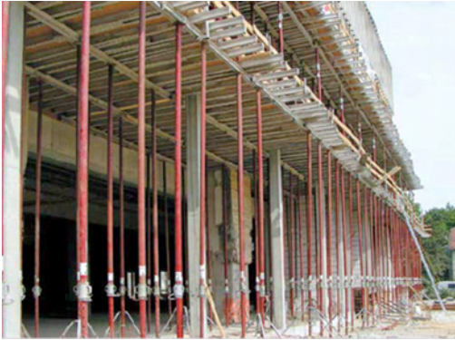
Fig. 3.1: Formwork for slab
