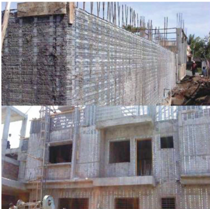
Coffor technology (Source: BMTPC)
