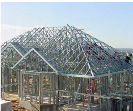
Fig. 6.3(a): LGS framing system
