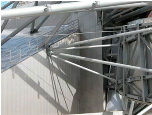
Fig. 6.18(e): HSS supports tying curved section
