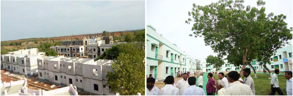
Fig. 4.20: GFRG building at Nellore, Andhra Pradesh
