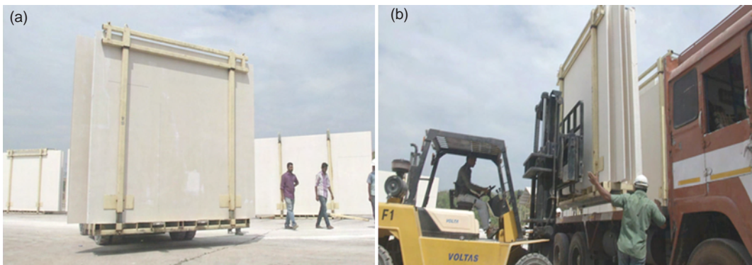
Fig. 4.6: (a) Panels stacked in stillages in the factory and, (b) loading of stillages on to trucks
