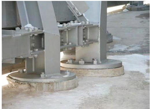
Fig. 6.18(l): Connection details of frames
