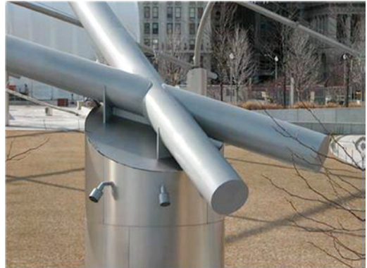
Fig. 6.18(n): Tube intersection connection
