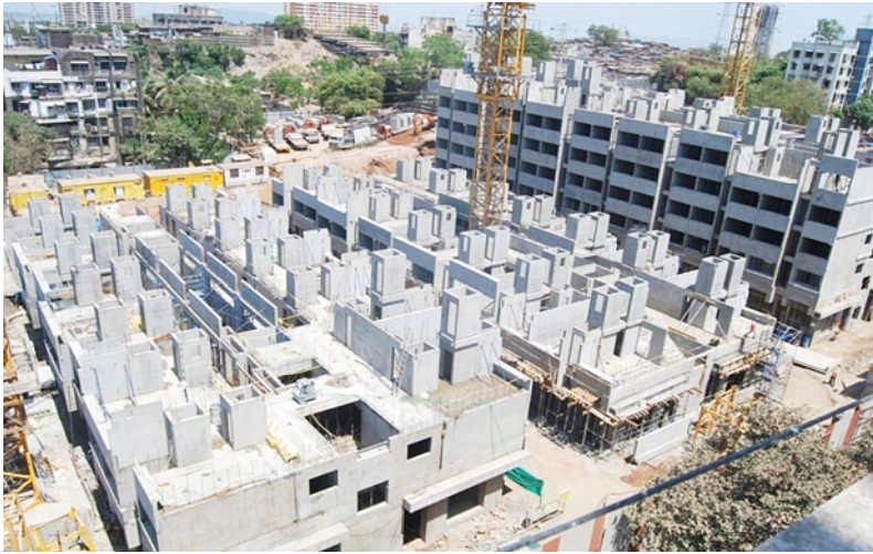
Fig. 7.3: Large panel system: High-rise apartment buildings at Mumbai
