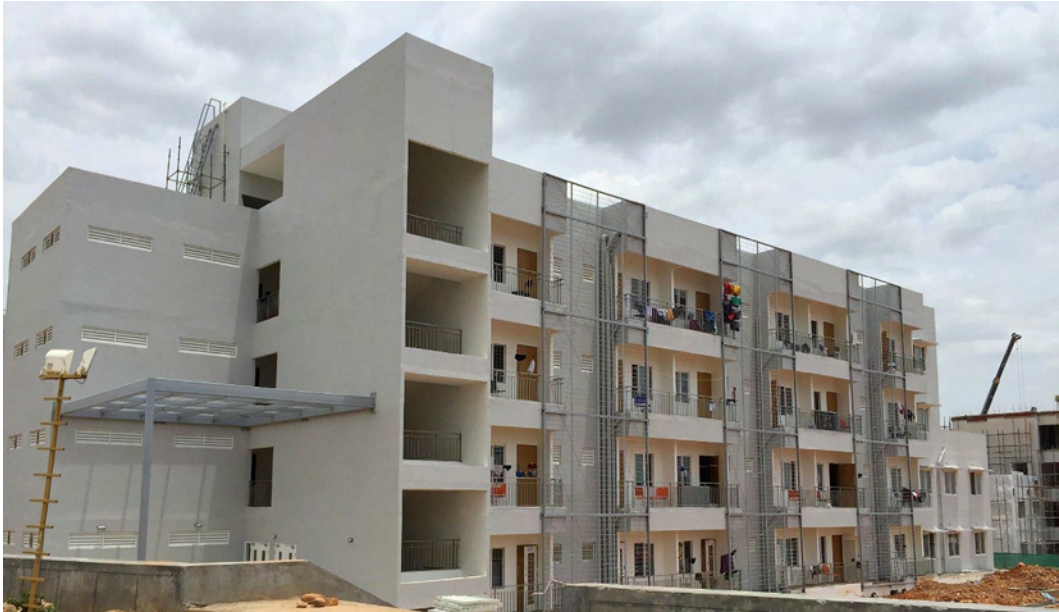
Fig. 4.23: GFRG hostel building (B1 block) at IIT, Tirupati (30,428.9 ft 2 )
