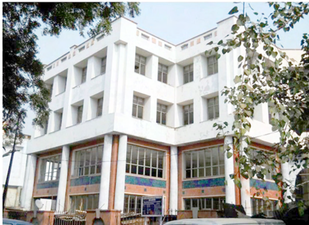
Fig. 6.14(a): Front view of the building
