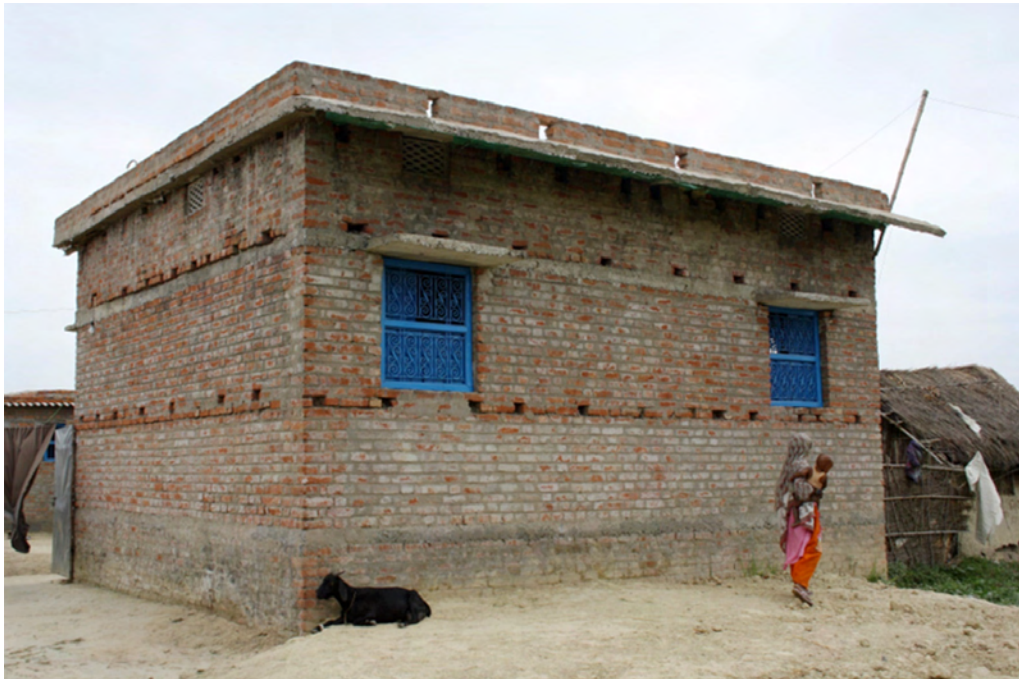
Fig. 1.4: Burnt clay brick masonry house
