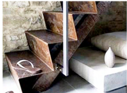
Fig. 6.9(f): Rusted steel finish stair
