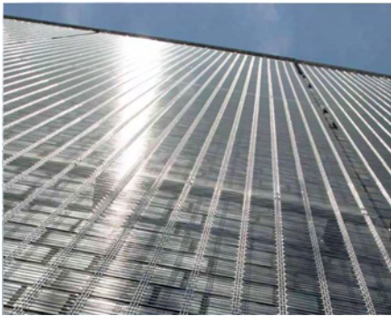
Fig. 6.6(c): Architectural mesh can be tensioned vertically over several stories
