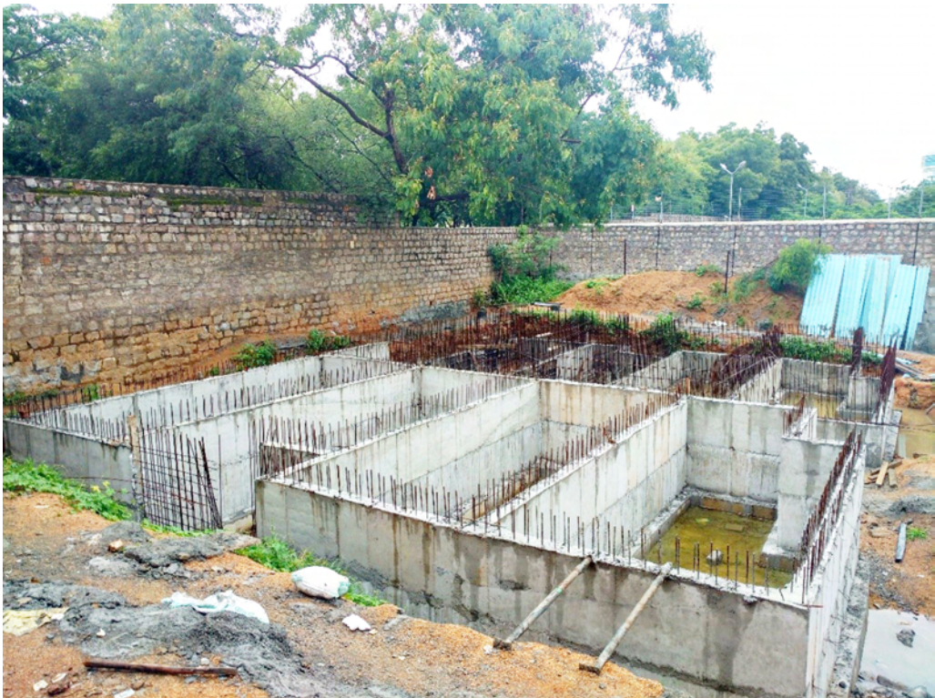
Fig. 6.5: RCC stem wall construction - completion
