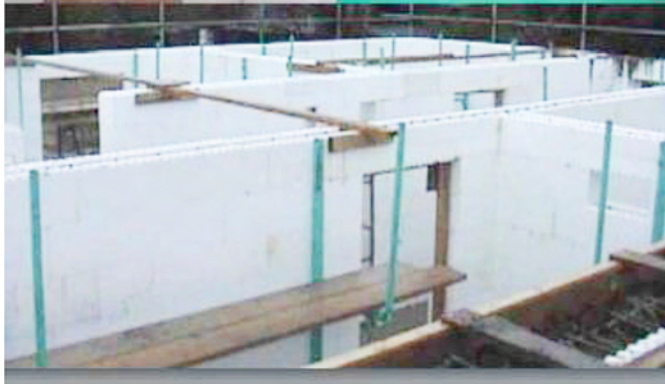
Monolithic insulated concrete system (Source: BMTPC)
