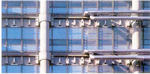
Fig. 6.17(d): The layers of structure, services and cladding articulate the elevation
