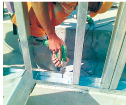
Fig. 6.4(b): Tracks used in LGSF
