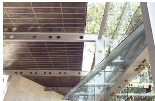
Fig. 6.12(b): Glass façade has spider joints supported by steel columns wraps over to merge with perforated steel ceiling panels
