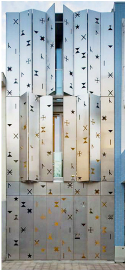
Fig. 6.6(b): Sensor controlled facades: controlling daylight and ventilation through foldable steel panel system
