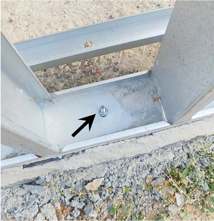
Fig. 6.8: Installation of LGSF frame can be done using mechanical anchor bolts (Courtesy: Hilti KB3 Expansion Anchor)
