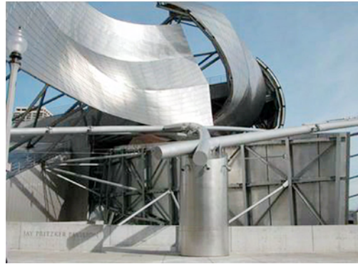
Fig. 6.18(d): Piers supporting HSS tubes
