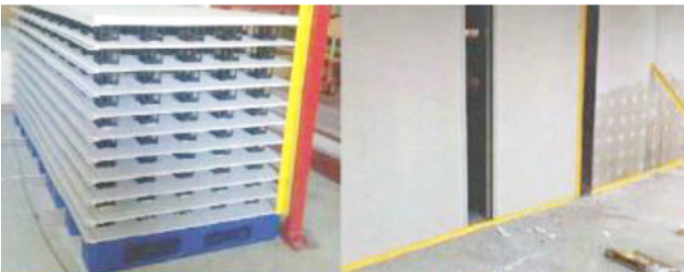
Lost-in-Place - Plaswall panel system (Source: BMTPC)
