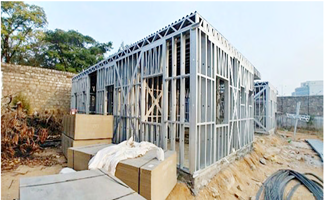
Fig. 6.11: Installation for floor deck panel for roof
