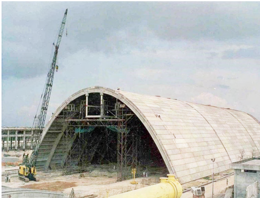
Fig. 7.5: Slab units on arches in a vaulted roof (Silo at Jagdishpur)
