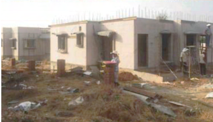
Lost-in-Place - Plaswall panel system (Source: BMTPC)
