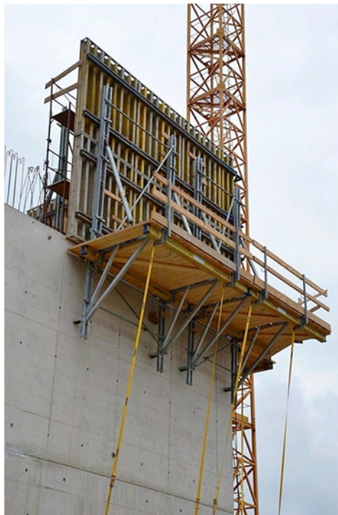
Fig. 3.3: Jump formwork
