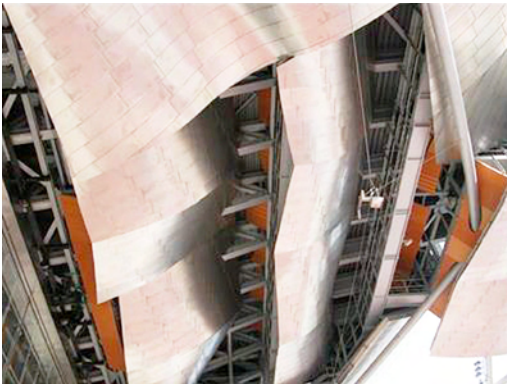
Fig. 6.18(k): Shell and truss support system
