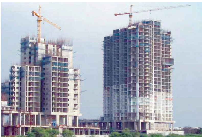
Fig. 1.6: Reinforced concrete frame construction
