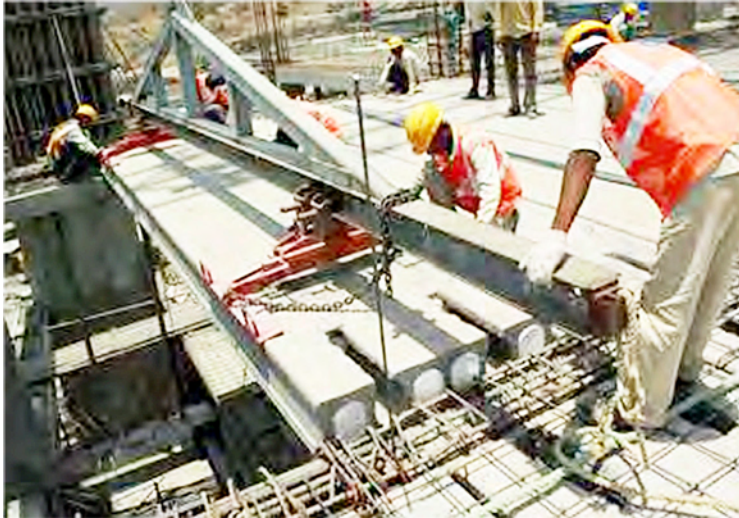
Fig. 7.7: Floors made of precast hollow core units (Canteen building, Pune)
