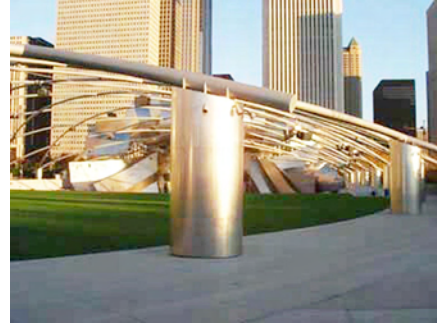
Fig. 6.18(b): Pylons supporting trellis
