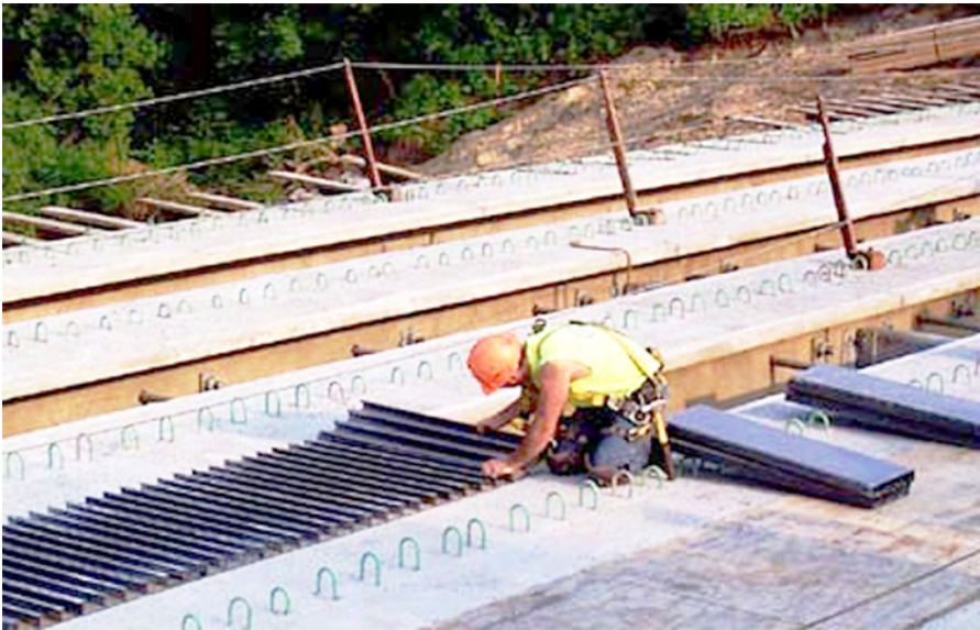
Fig. 4.19: Placing of FRP Planks between the girders [18]
