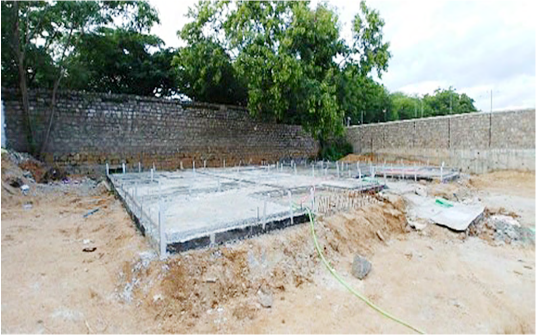
Fig. 6.6: Foundation platform for construction of LGSF structure
