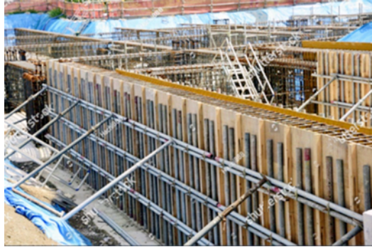
Fig. 3.2: Formwork for wall
