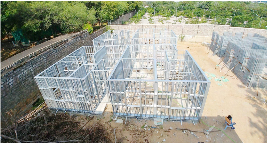
Fig. 6.9: Completion of LGSF frame for the ground floor
