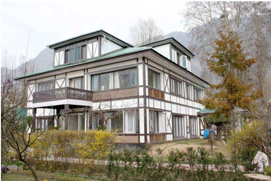
Fig. 1.2(b): Wood houses – Dhajji Diwari Houses
