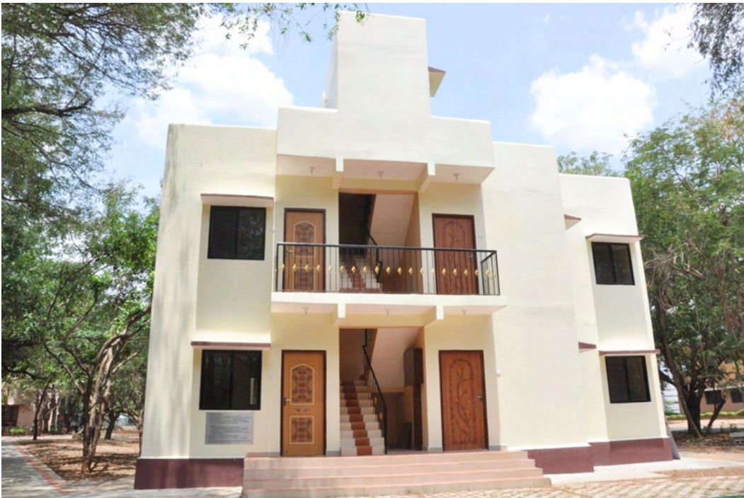
Fig. 4.18: GFRG demo building at IIT Madras campus
