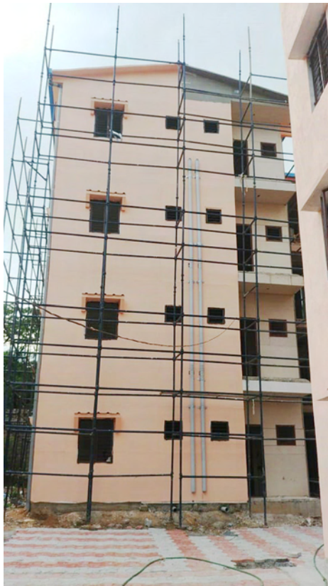
Fig. 6.15: View of the completed LGSF structure
