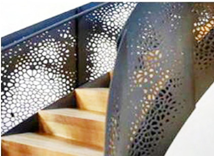
Fig. 6.9(e): Perforated steel balustrade
