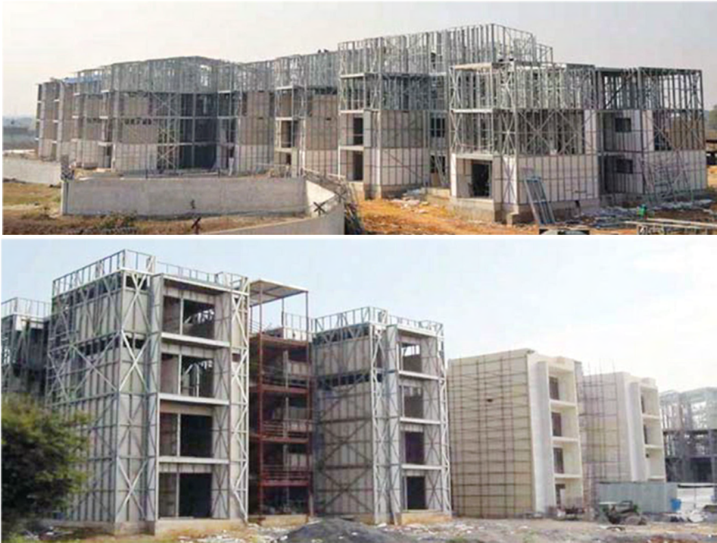
Fig. 6.5(h): LGSF building in different stages of construction
