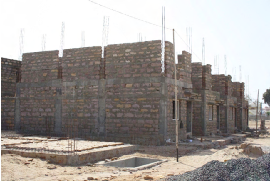
Fig. 1.5(a): Confined masonry house (under construction)
