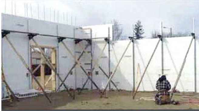
Insulating concrete form (Source: BMTPC)
