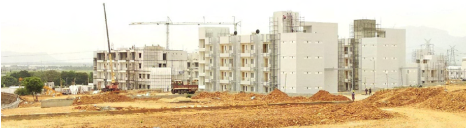
Fig. 4.22: GFRG hostel buildings at IIT, Tirupati (1.4 lakh ft 2 )
