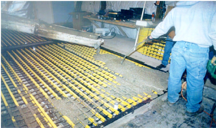
Fig. 4.14: FRP concrete deck preparation
