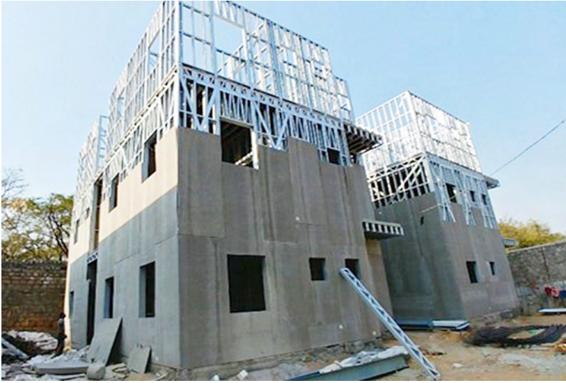
Fig. 6.14: Installation of sheathing boards (external cover) over LGSF frames
