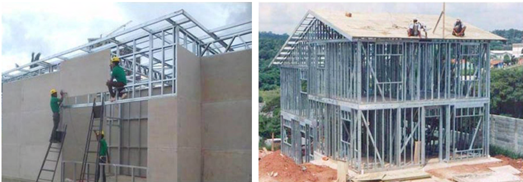
Fig. 6.5(g): Fixing of wall and roof cladding to LGSF
