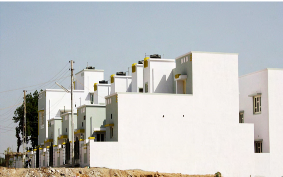
Fig. 1.5(b): Confined masonry house (finished)
