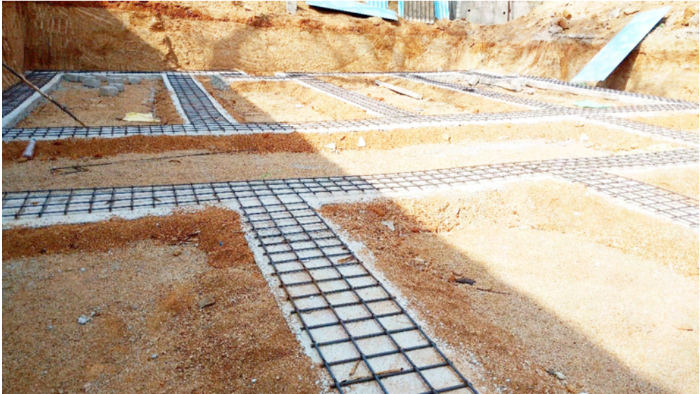
Fig. 6.4: RCC stem wall construction
