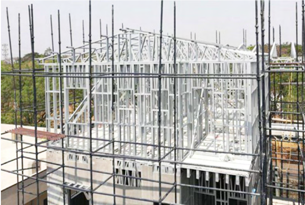
Fig. 6.12: Installation of LGSF frames for next floor
