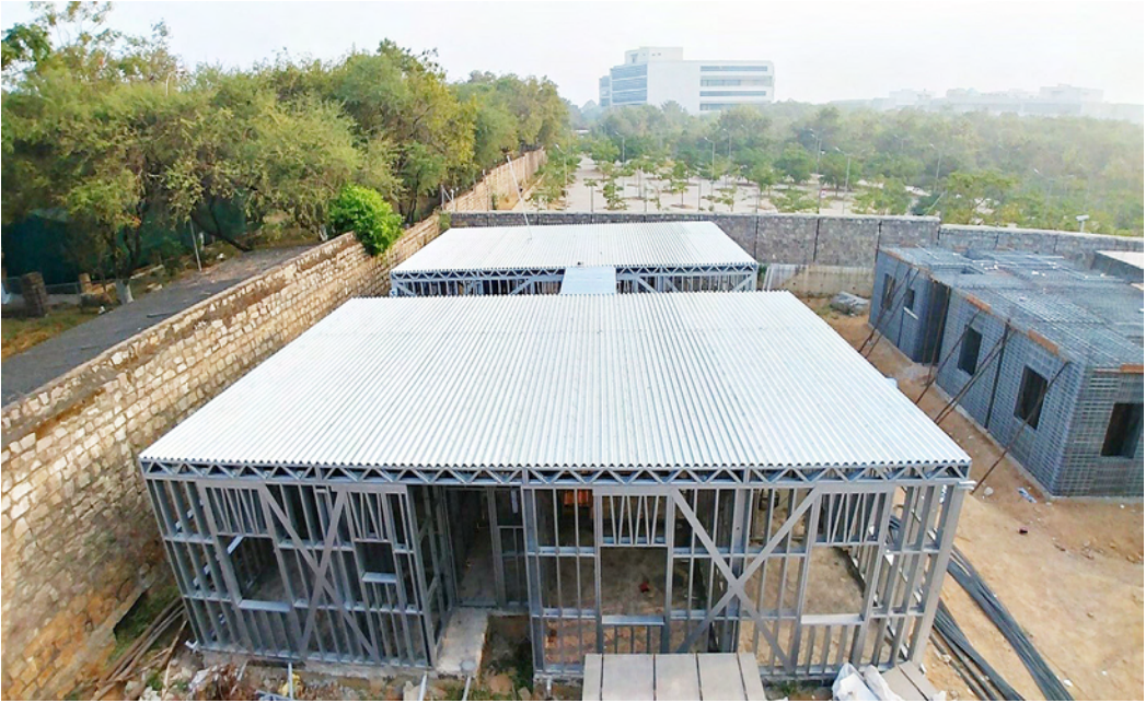
Fig. 6.10: Installation for floor deck panel for roof
