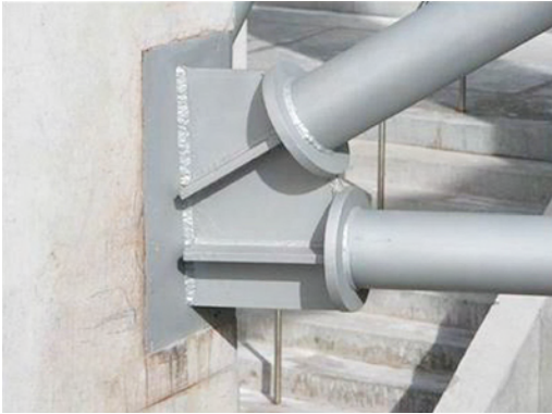
Fig. 6.18(i): Welding of steel
