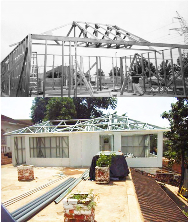
Fig. 6.5(d): Fixing of roof truss
