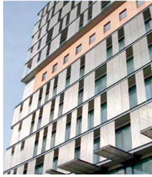
Fig. 6.6(d): Transparent architectural mesh elements combine sun protection
