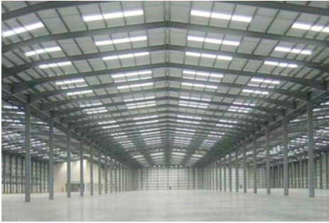
Fig. 6.2(a): Warehouse buildings
