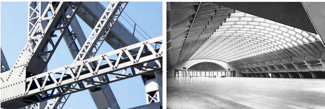
Fig. 6.7: Use of steel in infrastructure
