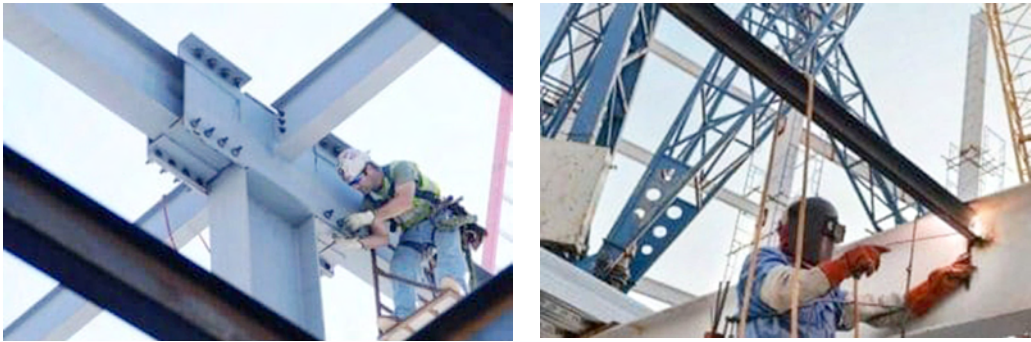
Fig. 6.3(b): Installation of LGS frames
