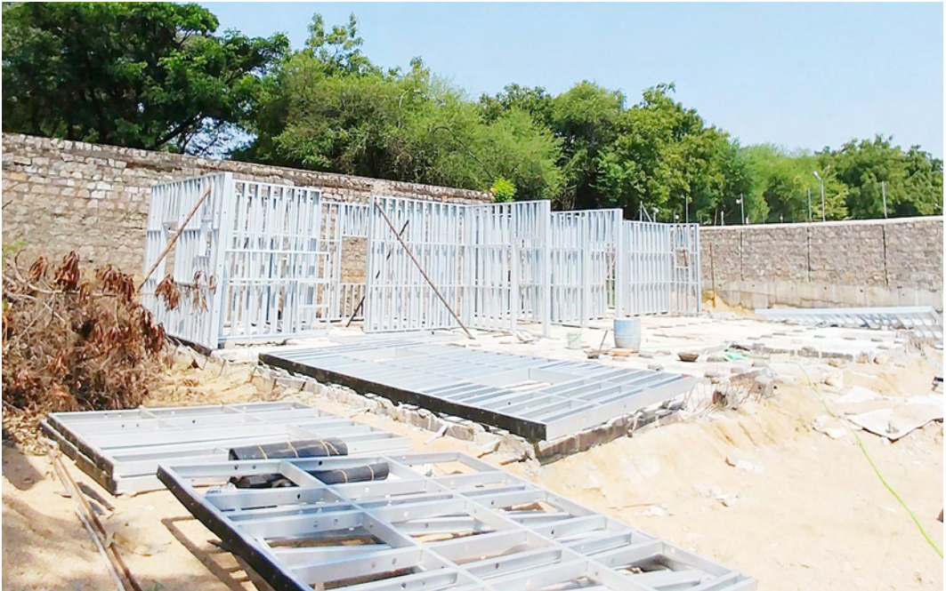
Fig. 6.7: Installation of LGSF frames
