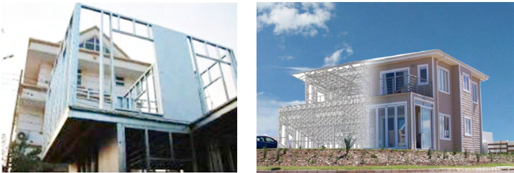
Fig. 6.3(c): House being constructed from LGSF
